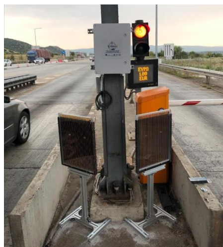
DSSC PV System Installation
