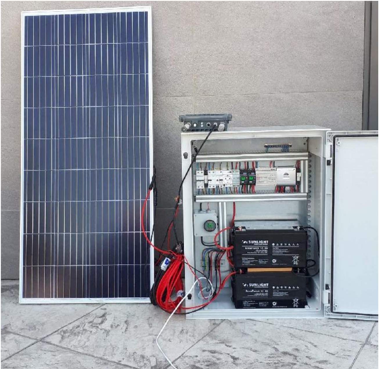
RSU Power Supply Control Panel
