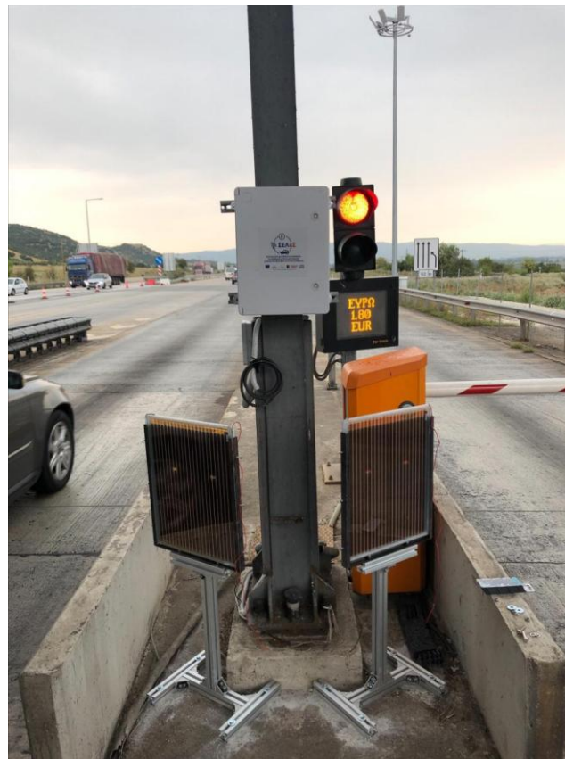
DSSC PV System Installation
