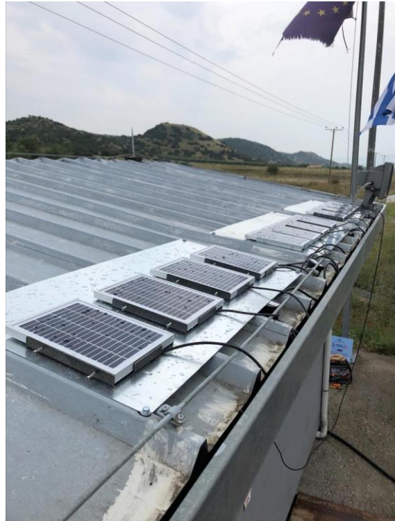
Conventional PV System Installation
