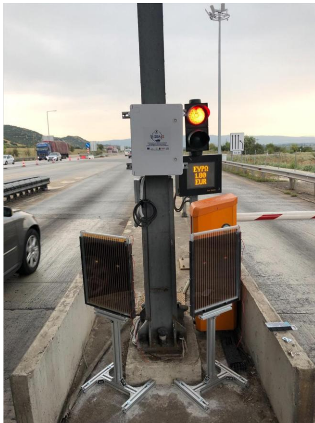
DSSC PV System Installation
