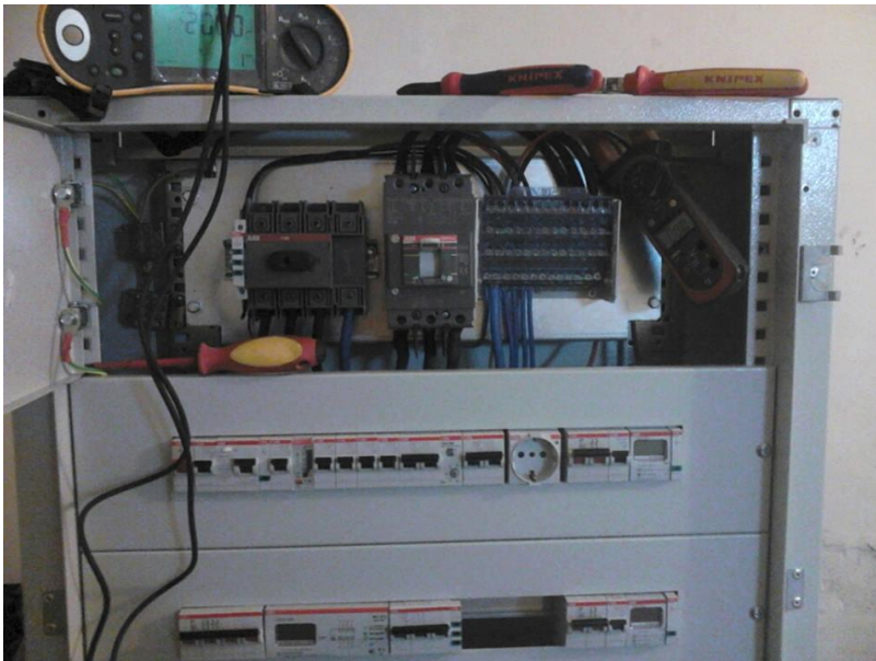
Electric Panel Inspection
