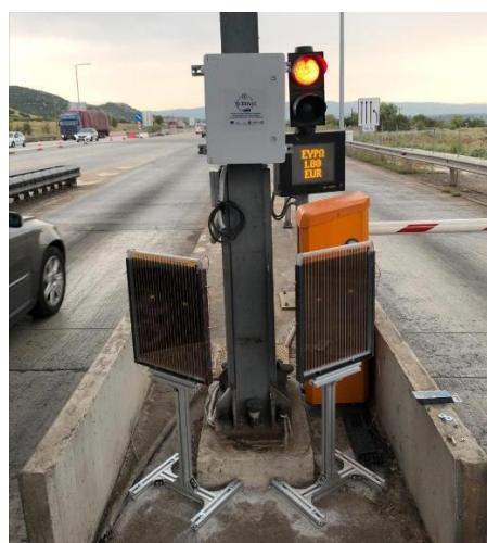
DSSC PV System Installation
