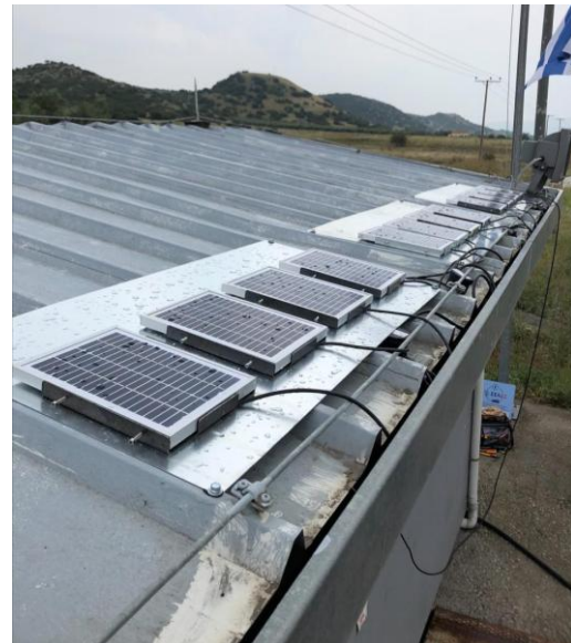
Conventional PV System Installation
