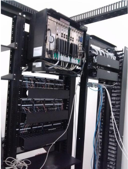
Telephone System Installation
