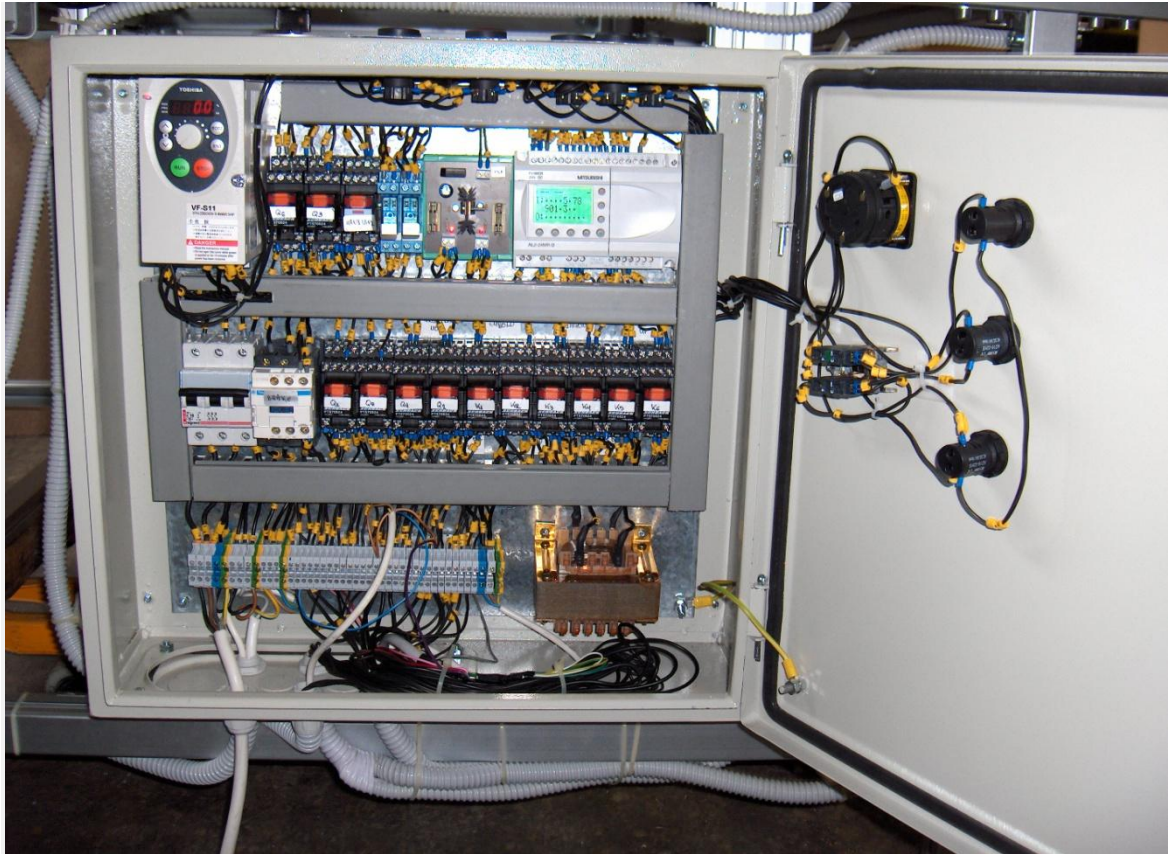
Electrical Panel Construction
