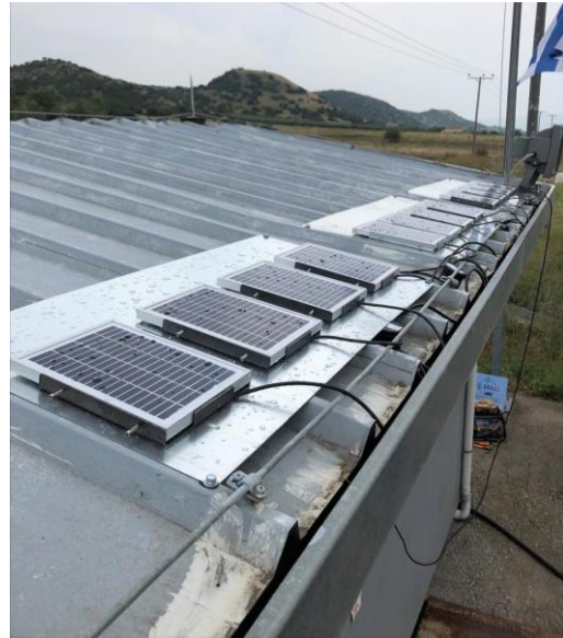
Conventional PV System Installation
