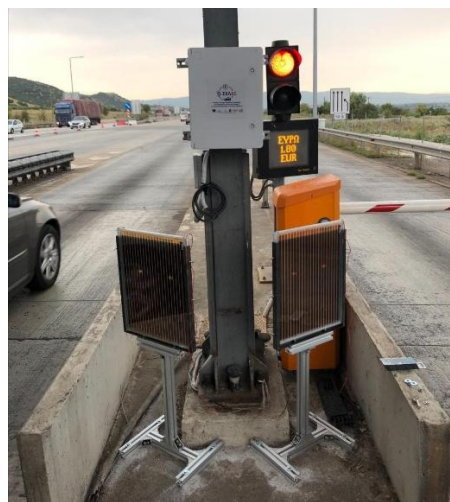
DSSC PV System Installation
